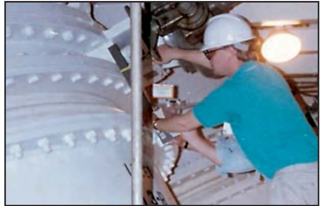
Fig. 2. Field measuring offsets and building replacement expansions joints to fit the application’s parameters not only minimizes installation time and expense, it ensures 100% of the joint’s allowable movement capabilities and operating life.
